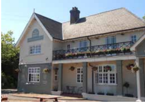
The White Horse refurbished
